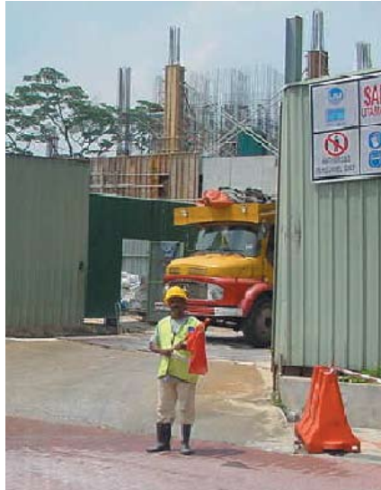
Entry to construction site
