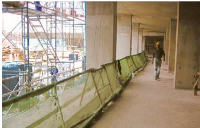
Walking through a building site
