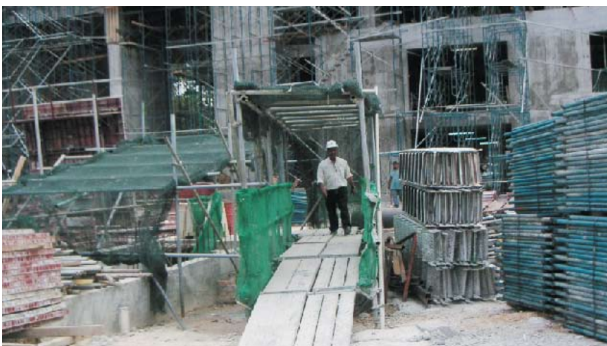
Contractor inspecting construction site
